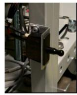
Panel Switch Installed - Bypass Mode Position
