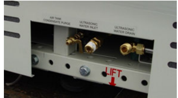
Figure 2-18 UCD Water Connections with Air Purge
