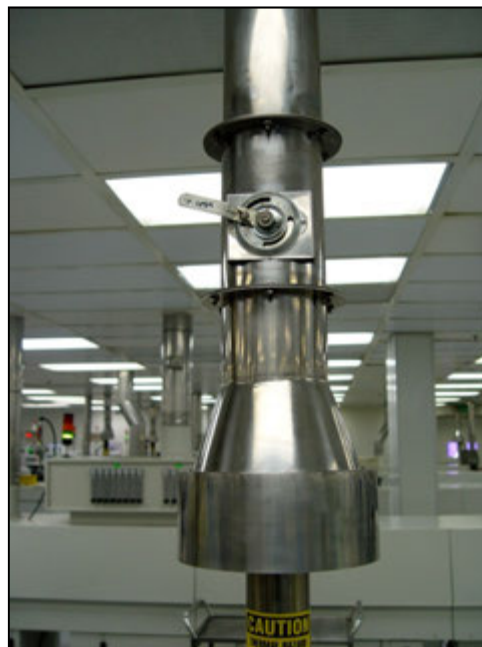
Figure 2-16 Exhaust Connection Detail
