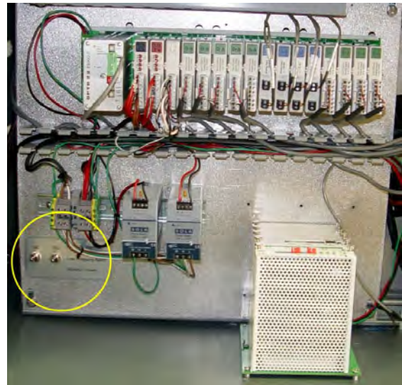
Figure 3-7 IPS Inlet Pressure Switch Location
